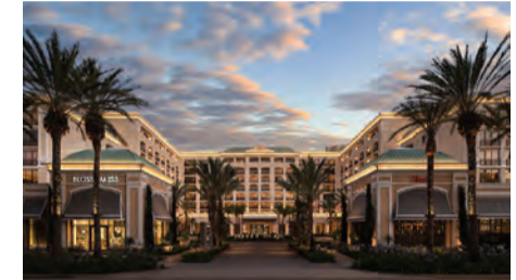
Project: The Westin Anaheim Resort Nominee(s): Wincome Hospitality Paul Sanford, CEO Wincome USA Kenneth Cheung, Director of Construction Larry Chu, Director of Engineering Judy Wang, Director of Purchasing Joshua Reitz, Development Manager HED Otis Odell, Principal, National Housing + Mixed-Use Sector Leader Michael Hong Architects Mike Hong, Design Principal KCS West Elmond Wan, President & CEO
